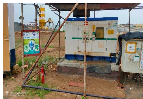
DG Set at Construction site
